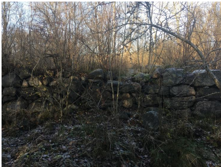
Figure 13, Stockby farm, Lidingö 59:1, close up of the foundation of what appears to have been the 19 th century farmhouse, Photo: George Wood
